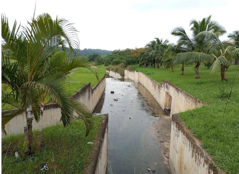
PLATE 1: Landscaping Protects Gully Control Structures in Uyo
